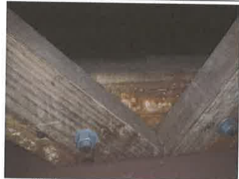
• Shows 100x50mm webs to 150x50 bottom plate connection
