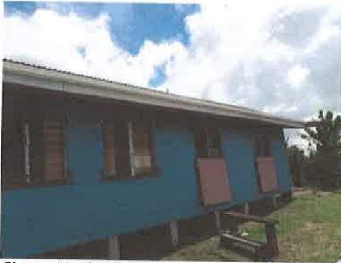
• Shows side elevation of inspected property.
