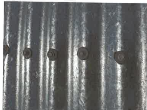
• Shows roofing screws currently used for roof fasteners
