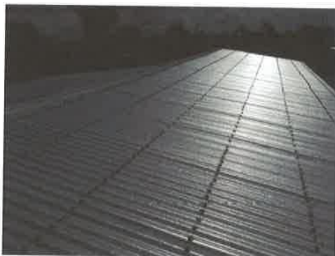
• Shows new roof cladding installed at the property
