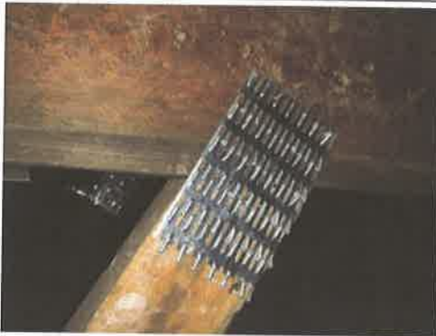
• Shows rafters to 100x50mm webs connection
