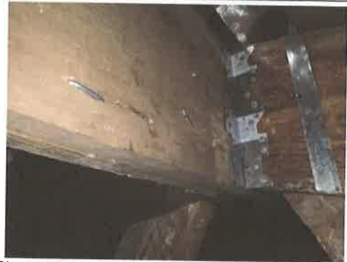
• Shows 150x50mm rafter connection to ridge beam
