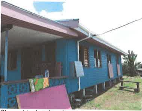
• Shows side elevation of inspected property
