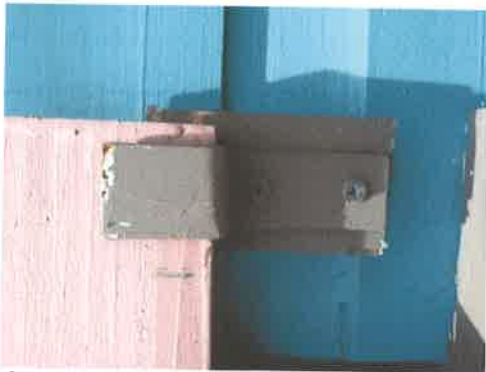
• Shows ply board shutter bracket
