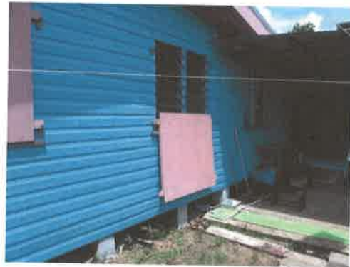
• Shows rear elevation of inspected property
